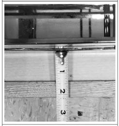
Measure 1-3/8" from behind face frame to the Slide Assembly (C).
