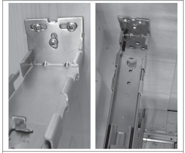
Remove the unit from the base again and then slide the rear mounting bracket off the slide. Align the rear bracket prongs with the indentation marks on the rear of the cabinet and secure with three (3) #8 x 5/8" Pan Head Wood Screws in the slots as shown. Re-install the unit onto the slides, making sure as you push it in the cabinet, that the top slide is properly seated into the rear mounting bracket. Operate the unit to make sure the undermount slides are working properly.
