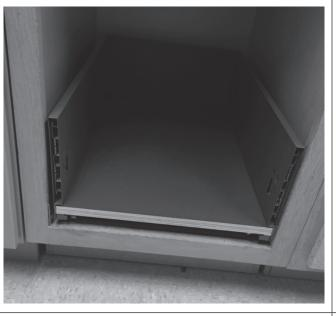
Place the metal drawer box inside the cabinet and slide it on the slides to the end until a click sound is heard.
