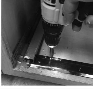
Install the slides with the metal runners inside the cabinet using the screws provided according to the pictures above.
